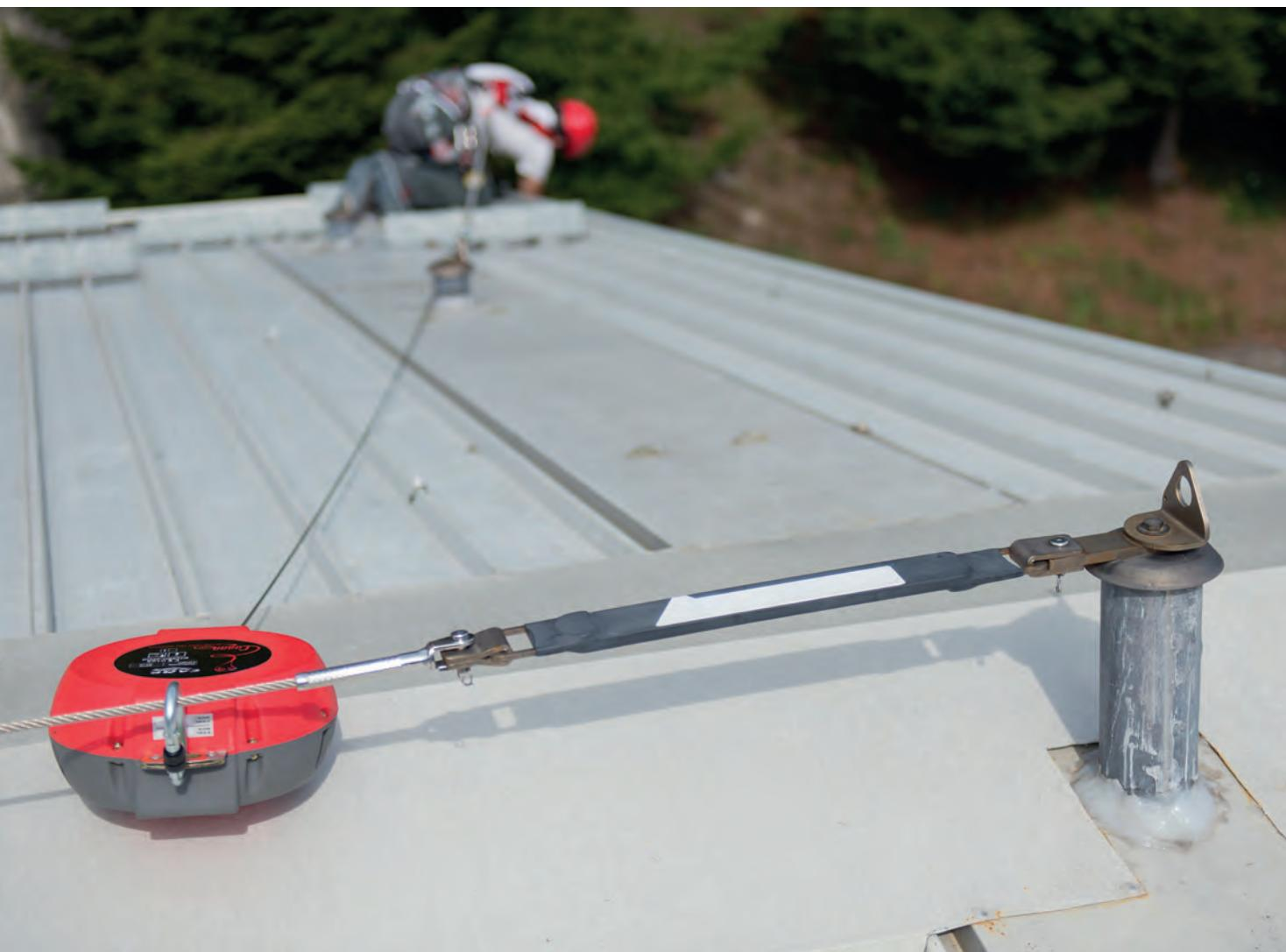
The Cobra 10 retractable device being used in the maintenance of a roof.
